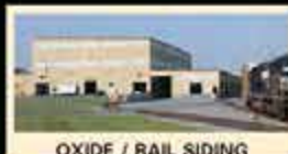
OXIDE / RAIL SIDING
