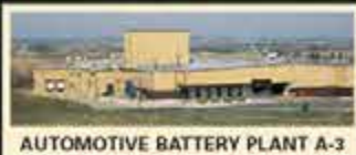
AUTOMOTIVE BATTERY PLANT A-3
